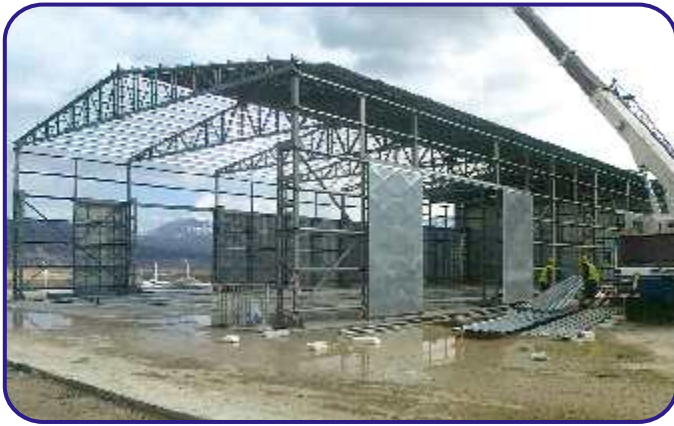
Depo Hangar Binaları / Large Store Building
