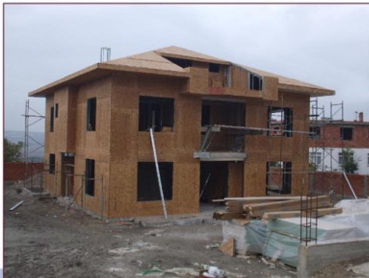
Light steel constuctions can easily be disassambled with low loss of material and can be assmbled again somewhere.
