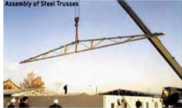
Assembly of Steel Trusses
