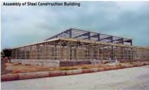
Assembly of Steel Construction Building
