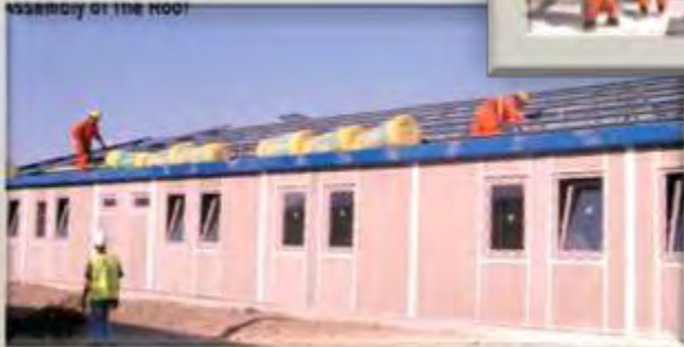
assembly of the roof
